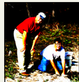
Bernie and Roy hard at work on waterline repair
